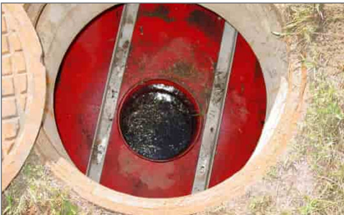
Fig.7 View over center shaft into sediment storage zone.
