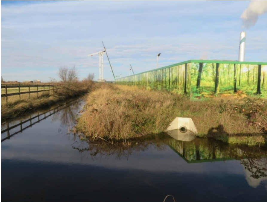
Photograph 2.1: An existing outfall from the compound into a ditch on the western and southern side of Borax North.
